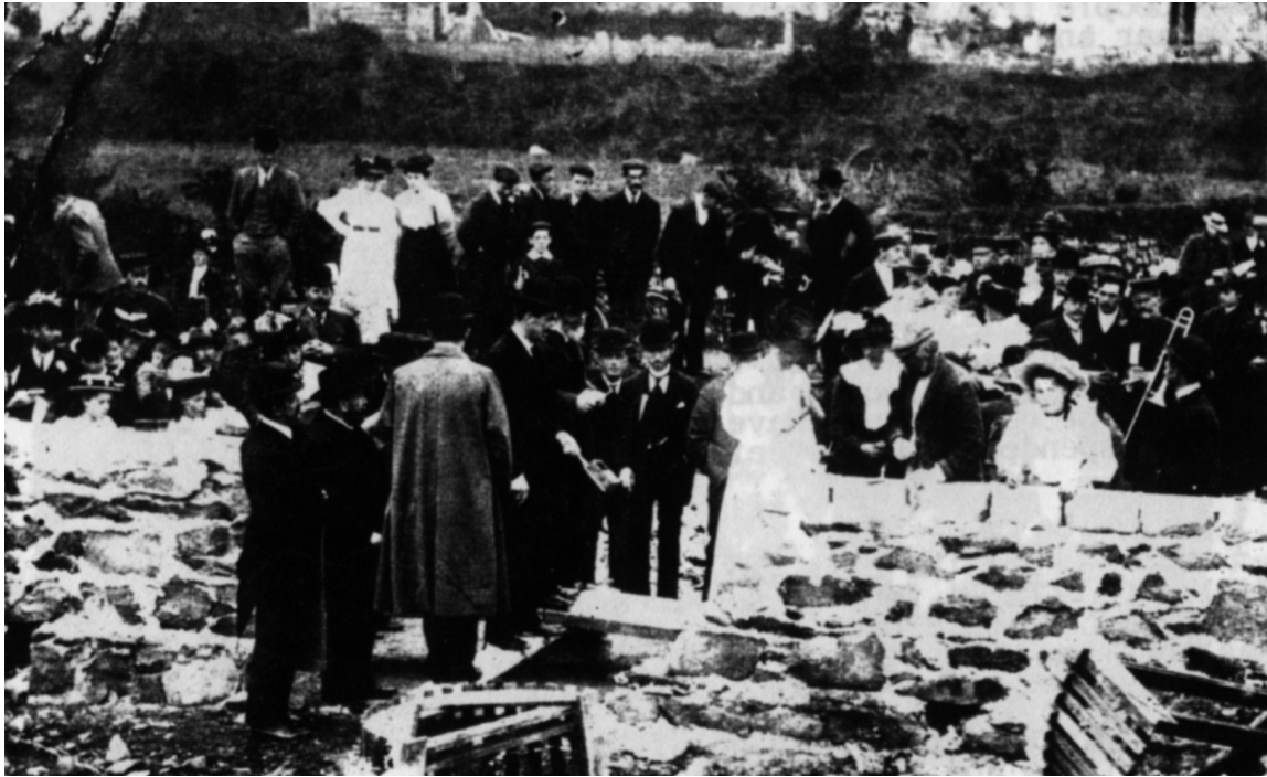
2. Stone laying - new chapel. 1907
